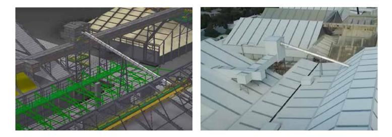
Our client was re-developing their site in Christchurch after the 2011 earthquakes. As part of the upgrade, the intake system required replacement along with the affected buildings. We were commissioned to design, fabricate, and install a fully enclosed, 400 TPH, long span air-supported belt conveyor to transport various products into the bulk storage buildings on site.
